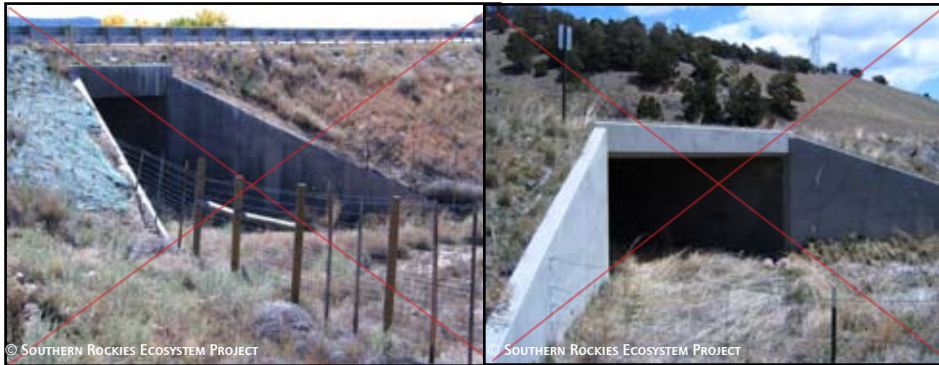
EXAMPLE OF GOOD FENCING THAT TIES INTO THE TOP OF A CROSSING STRUCTURE: MULTI-PLATE ARCH ON US HIGHWAY 40, BERTHOUD PASS, COLORADO (TOP). EXAMPLES OF POOR FENCING: CORRAL EFFECT FENCING ON US 550, NEW MEXICO (BOTTOM LEFT), LIVESTOCK FENCING BLOCKING AN UNDERPASS ON HWY 50 IN COLORADO (BOTTOM RIGHT).
